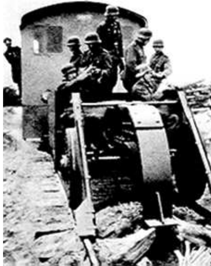
The "Rail wolf" pulled by a locomotive rips the rail sleepers like matches.
